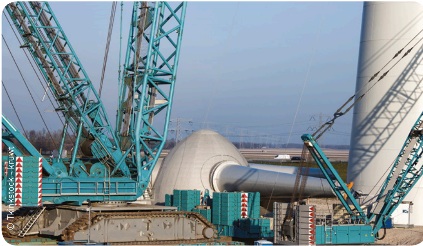
Assembly of wind turbine
