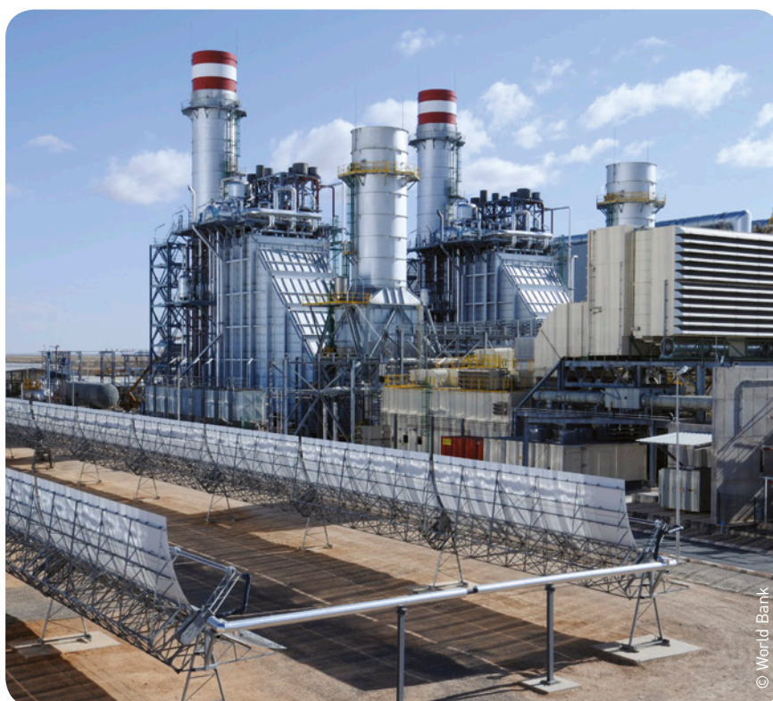
Thermo-solar power plant in Ain Beni Mathar, Morocco
